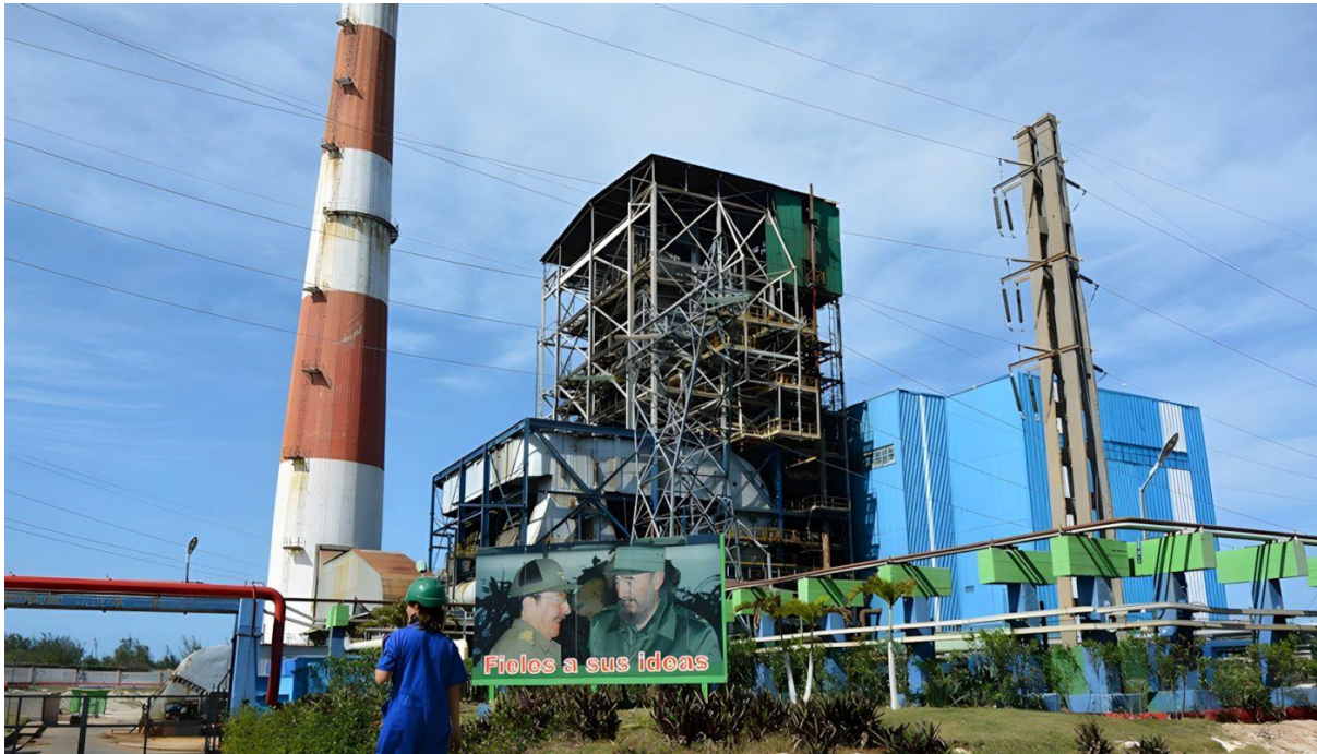
The Antonio Guiteras power plant in Matanzas, built in 1988 (KI-scaled) (Source: Cubadebate )
